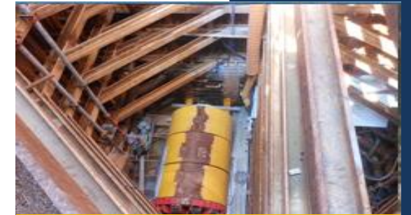
TBM in Jacking Pit at 25m depth below ground level
