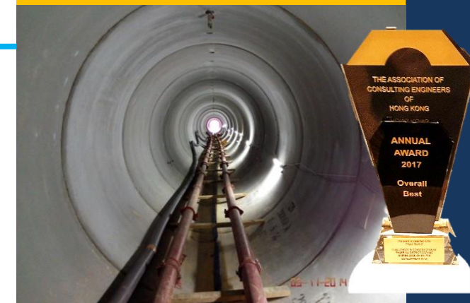
Subsea Tunnel (350m) at Kai Tak Approach Channel
